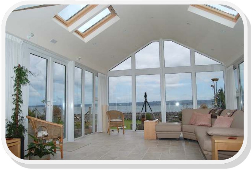
An extension with tiled roof and Velux roof lights Giving panoramic views of their surroundings
