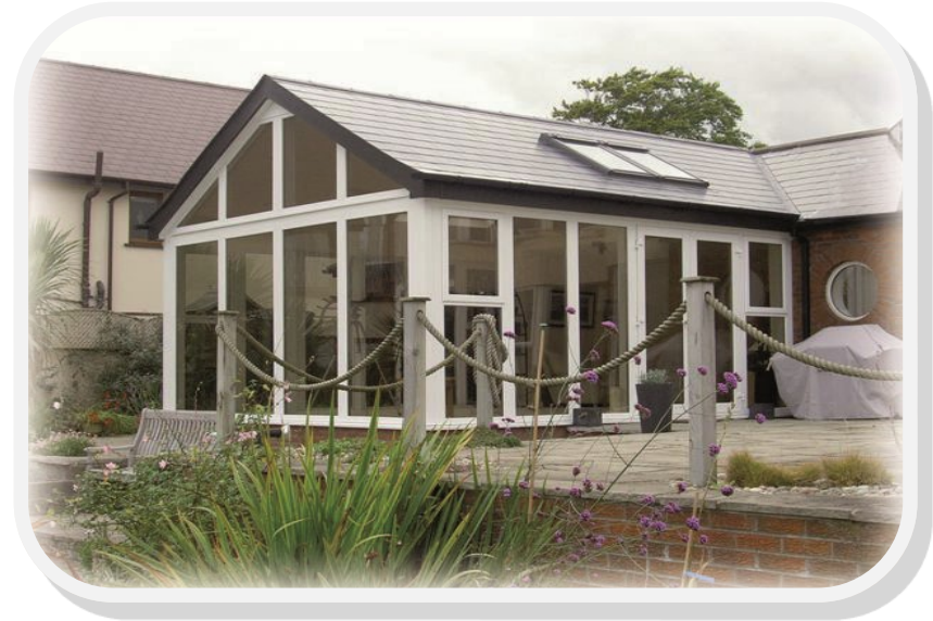
The roof can be finished with slate or tile in a size and colour to compliment your existing home
